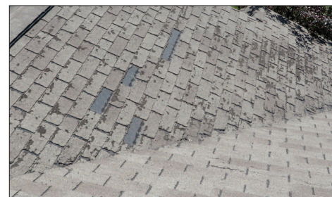
Lake Orion Roofing finds hail damage after inspecting the integrity of this homeowner’s roof. Damaged shingles are not as effective in protecting the home from further leaks.
